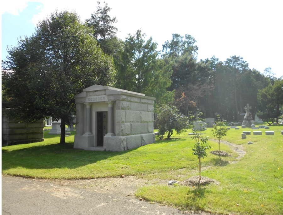
Figure 4 10 : Georger Mausoleum in Existing Landscape (Crabapple Tree to the left, Rhododendron Tree to the right)
