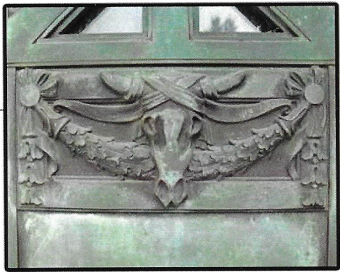
The door is made of bronze, as are the air vents for the mausoleum, and the frame for the stained glass window found on the east side of the building. The bronze has a patina which is protecting the bronze, keeping it in fine condition and lending a pleasant aesthetic value to the design.
