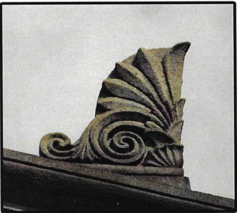
The acroterion is a typical example of the ornamentation found in other buildings designed by McKim, Meade, & White. These few ornaments show that Sherry, though wealthy enough to afford the services of the firm, was not ostentatious. Instead, the design for his resting place is tactful and elegant.
