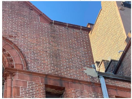
Figure 8. Damage to masonry on east facade (Photograph by author, 2021.)
