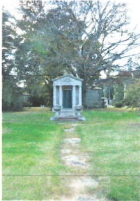
view from road (56' from mausoleum)
