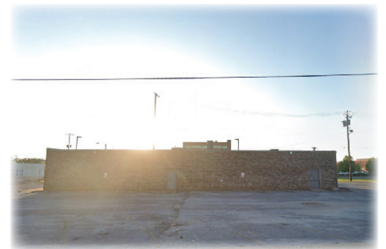
Current view of the site
