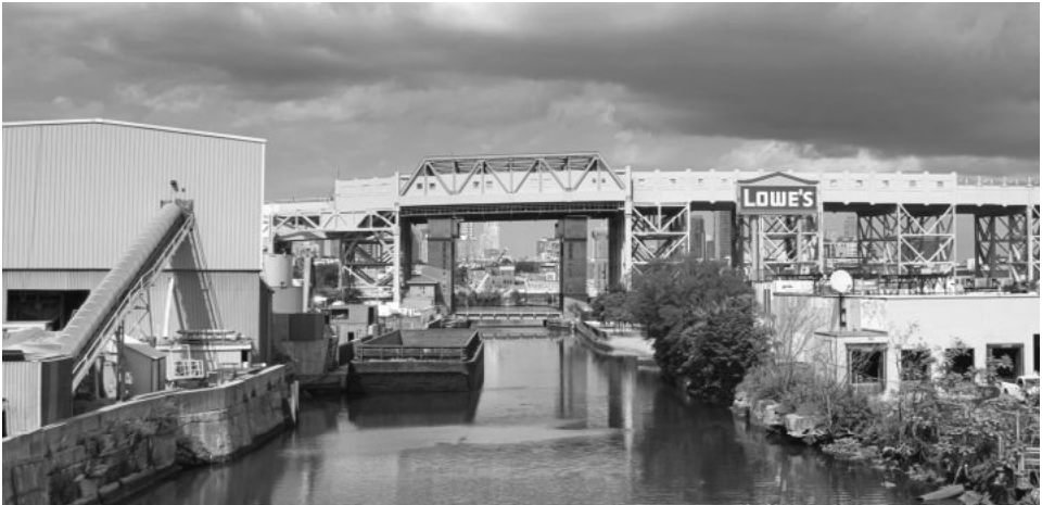
Smith-9th St Station before renovation
