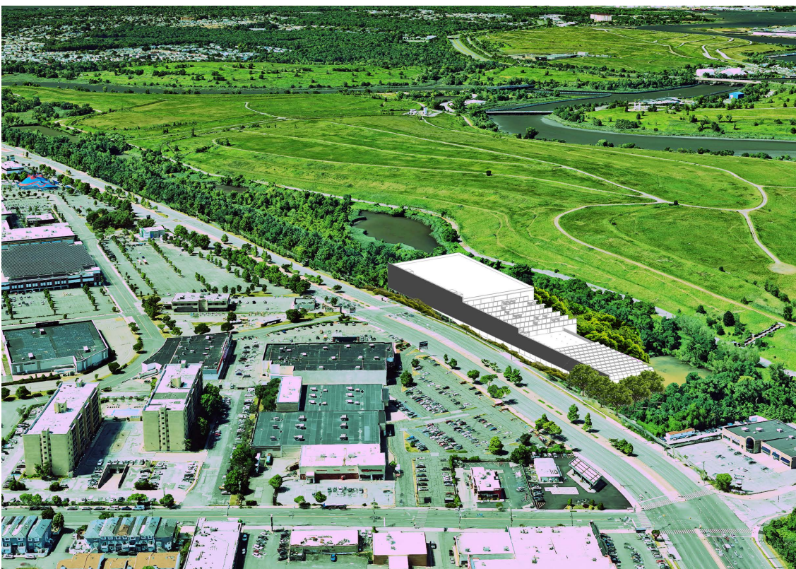
Collage of the exterior of the building in the surrounding area, Freshkills Park on the right, the neighbourhood on the left.
