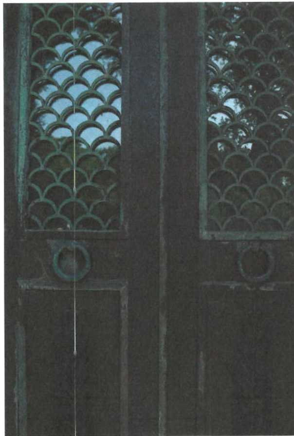
Figure 5. The green patina starting to form around the edges of the bronze door
