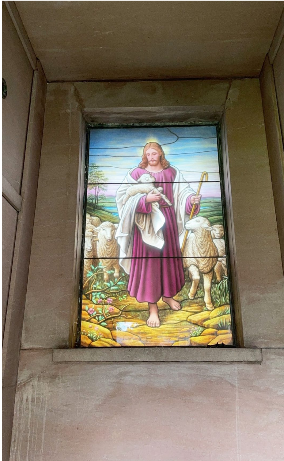
Figure 9: Stained Glass Detail and Documentation of Water Damage around Joint Lines
