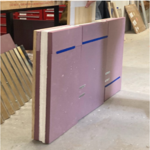
Applying sheathing to insulation and air-vapor barrier
