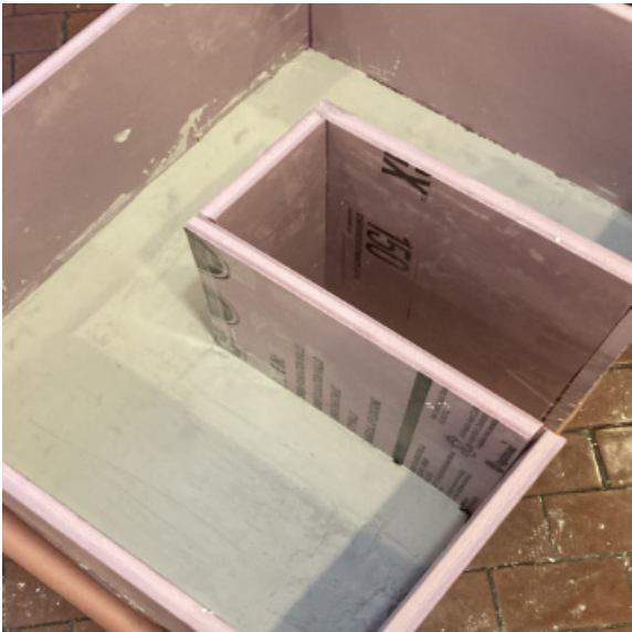
Pouring the concrete topping over the CLT
