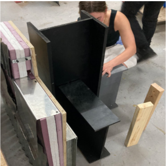
Attaching wall assembly to structure
