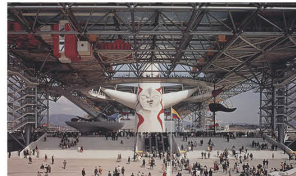
Figure 1. Kisho Kurokawa's Capsule House installed inside the space frame of Kenzo Tange's Big Roof, suspended thirty meters above the festival plaza.
