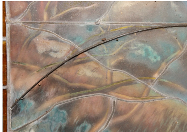
Figure 10. Photo of detached horizontal bar (third from top) on Gethsemane window.
