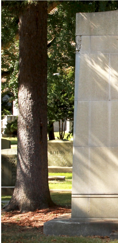
Figure 1. Photo of chamfers on the Wallace mausoleum.
