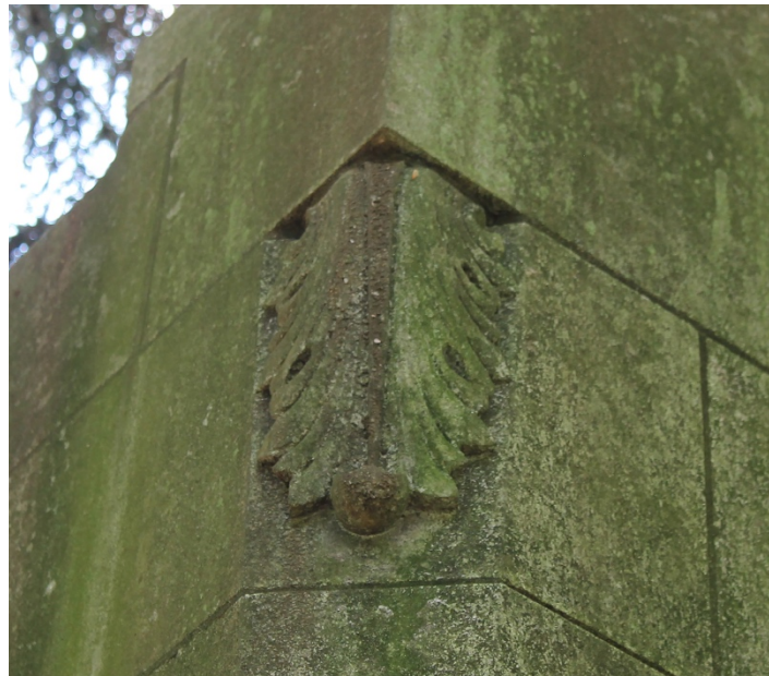
Figure 2. Photo of acanthus leaf chamfer stop.
