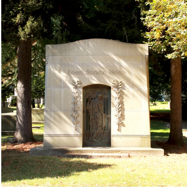
Figure 13. South (primary) façade.
