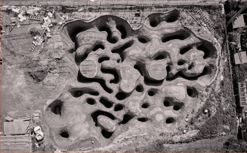
fig 1: Construction Photo of the Ube House Source: Architectura Viva
