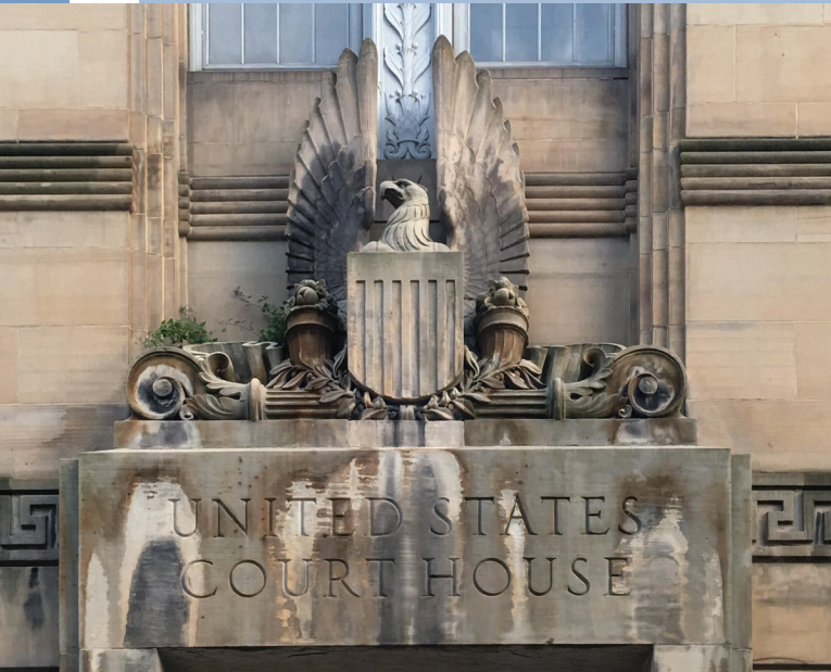
The facade of the historic Dillon Courthouse, a federally owned building that helped kick-start Buffalo's recent film renaissance.
