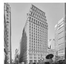
Existing Office Building 550 7th Ave
