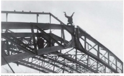
From the site of the New York State's expressed intention and... October 1910, officially designated as the 1908 Field Armory. The... On 10 August 1914, the Eighth United States Cavalry was... The unit was converted into a mounted field artillery unit and, on 11...
