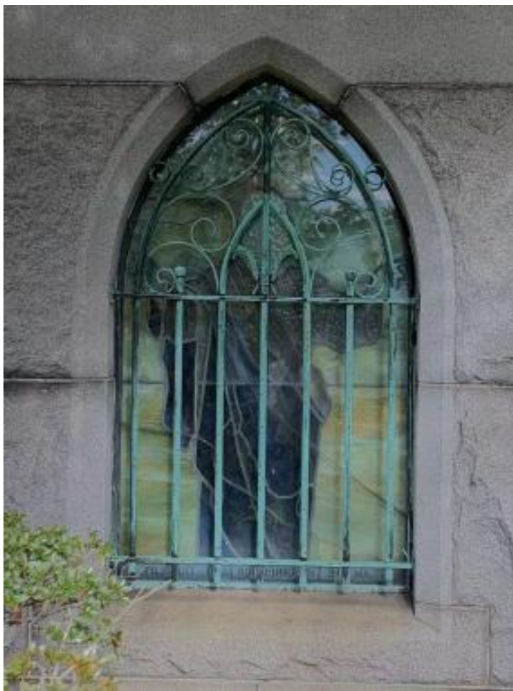
Fig.4 The granite around the windows imitating an outer window frame
