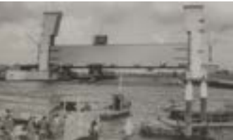
The storm surge barrier under construction, completed in 1958 1
