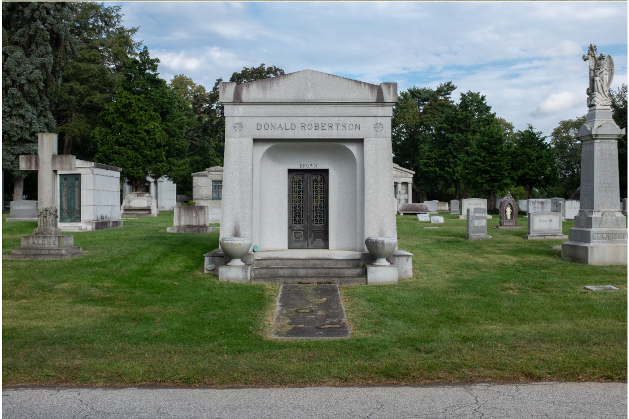
Figure C & D: Robertson Mausoleum (south elevation and facade)
