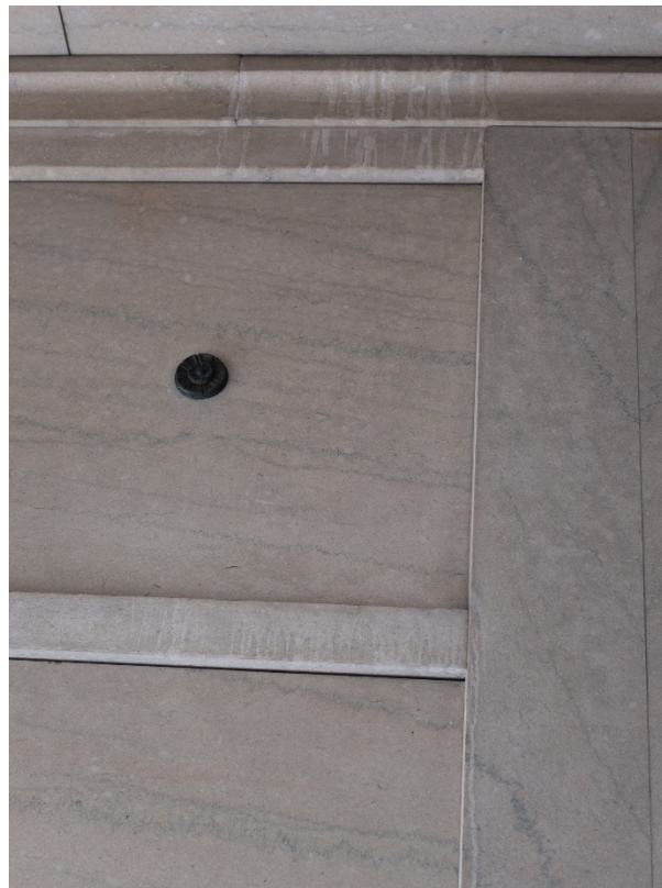
Figure H: Interior water damage (northeast corner)
