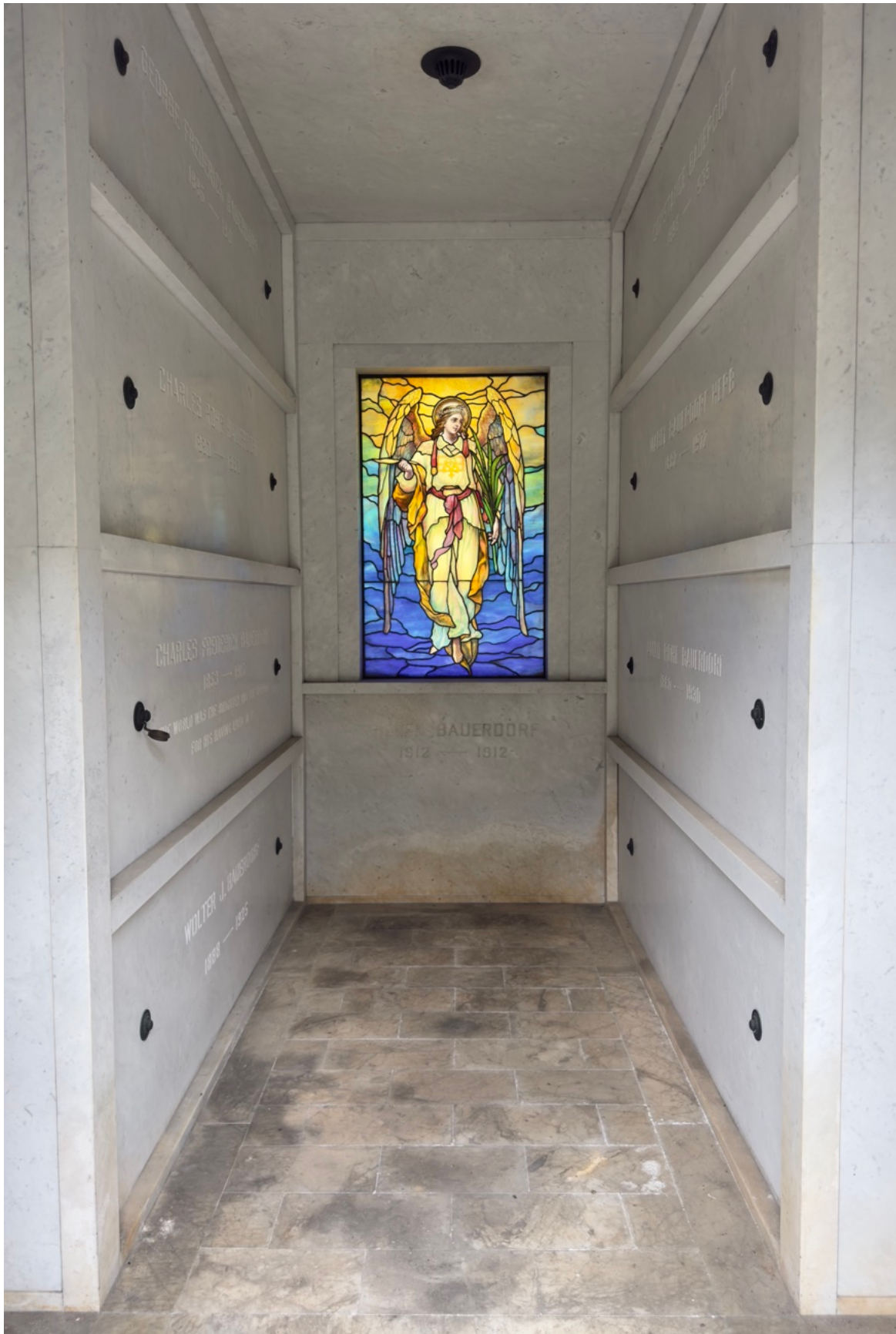
Figure 7. Interior rear looking west.
