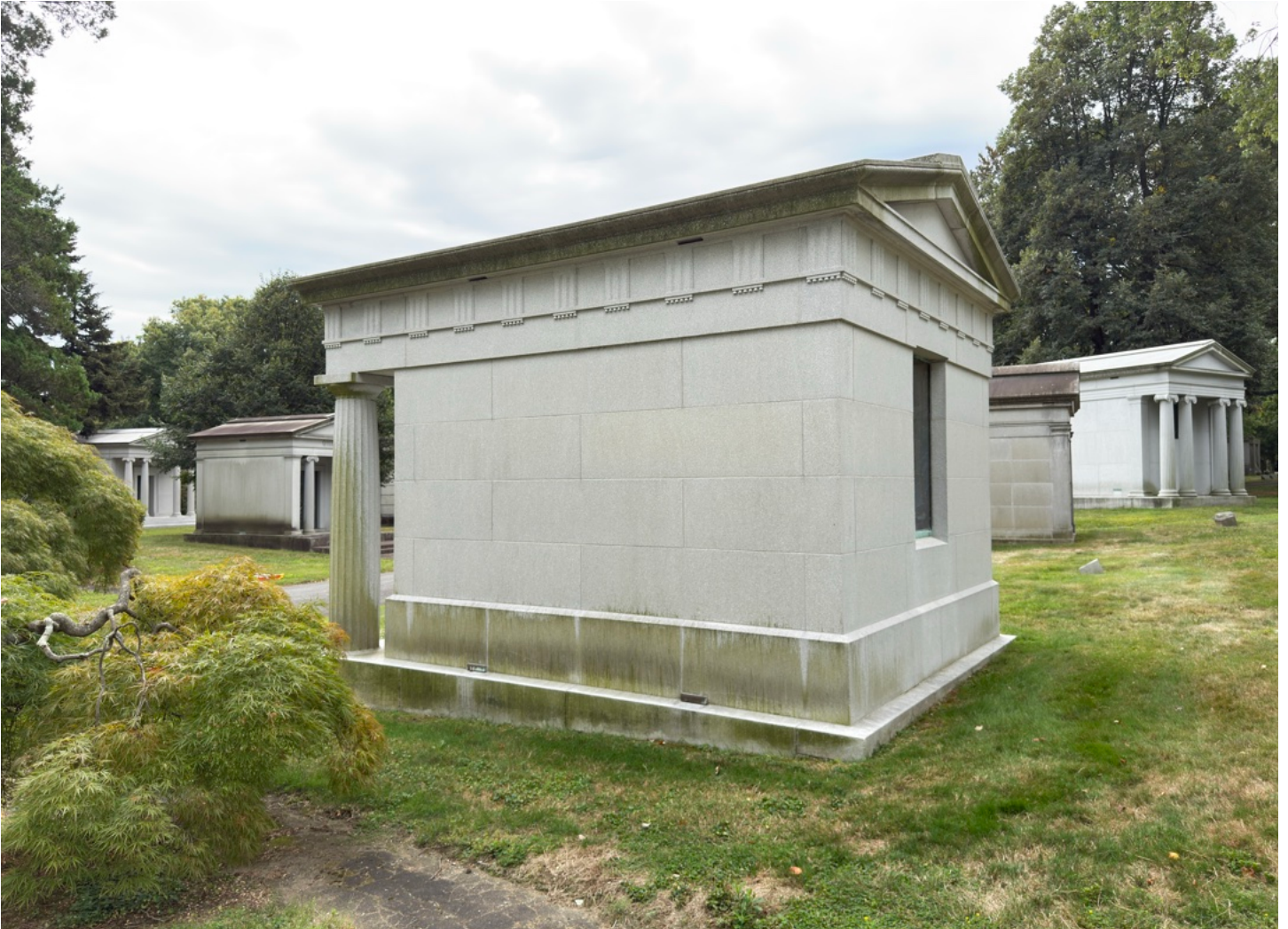
Figure 6. Side elevation from the north.
