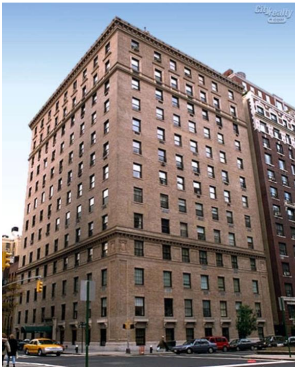
The Norma 960 Park Ave., New York, NY. Built 1912, converted into a cooperative in 1915. -Photo by City Reality
