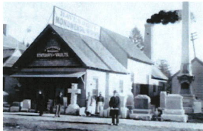
jerome ave. havender's monumental works during operation (c. 1903) (john mcnamara collection)
