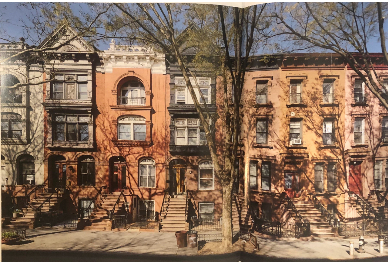
Figure 4. The houses at 10-18 Arlington Place, Bedford-Stuyvesant, Brooklyn
