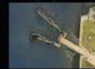
Ferry Dock Material: Concrete, Steel and Timber Status: In Use
