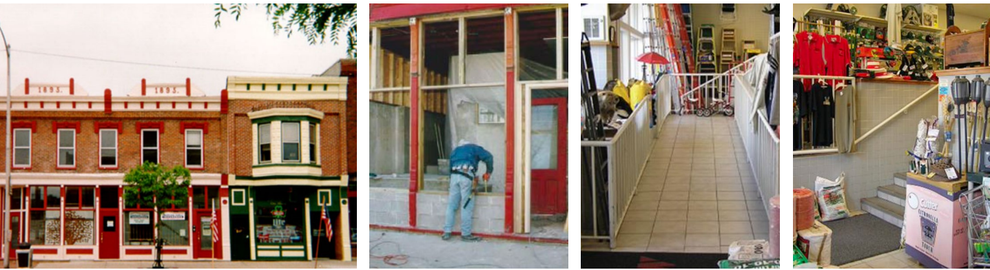
Successful Case: Non-structurally elevated storefronts in Darlington, WI. Source: FEMA 2008, 17; Nantucket 2021, 65–67.
