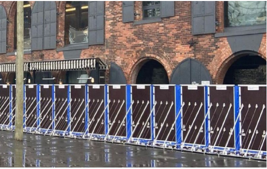
The Deployable Flood Shield System Protecting the Empire Stores. Source: Twitter Posting of AquaFence .
