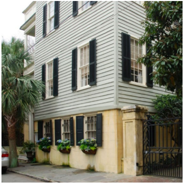
Solution 2 | Adaptively Articulated, Solid Foundation Walls. Sources: Photograph taken by the author during Keeping History Above Water 2021 Conference; Charleston BAR 2019, 5.
