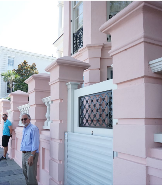
A detached residence with dry-floodproofing perimeter walls in Charleston, SC. Source: Photograph taken by the author during the Keeping History Above Water 2021 Conference.
