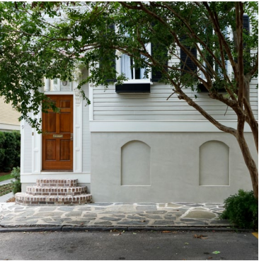
Solution 2 | Adaptively Articulated, Solid Foundation Walls. Sources: Photograph taken by the author during Keeping History Above Water 2021 Conference; Charleston BAR 2019, 5.
