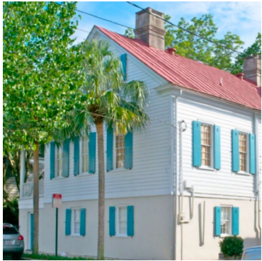
Solution 2 | Adaptively Articulated, Solid Foundation Walls. Sources: Photograph taken by the author during Keeping History Above Water 2021 Conference; Charleston BAR 2019, 5.
