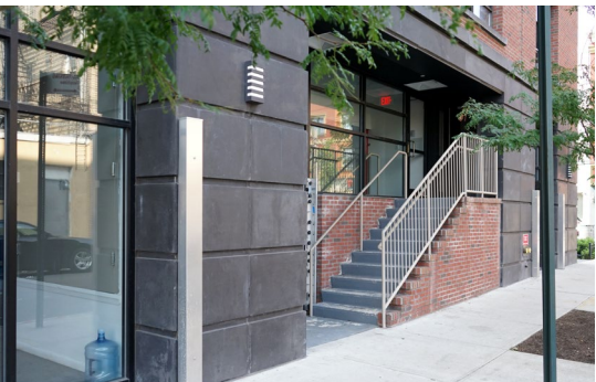
Permanent egress above DFE in a newly-built mixed-use building in Staten Island. Photograph taken by the author.
