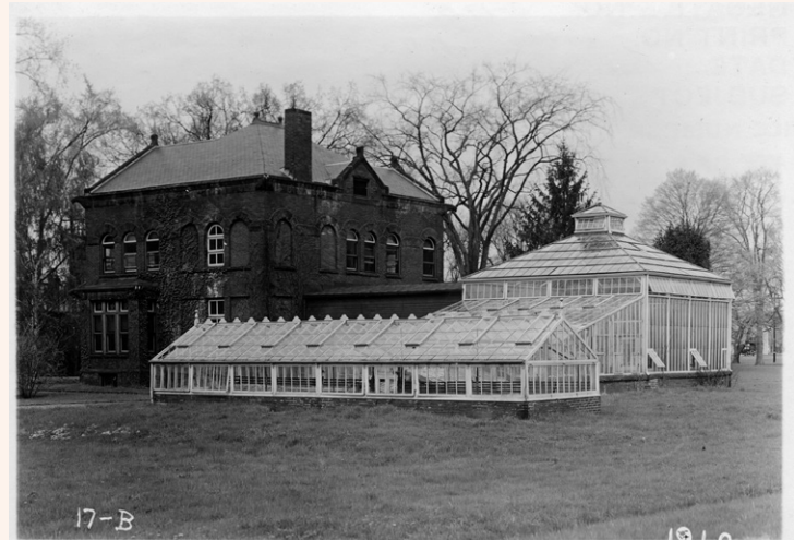
East Experiment Station, view of the rear of the building with greenhouses, 1918. Special Collections and University Archives, University of Massachusetts Amherst Libraries
