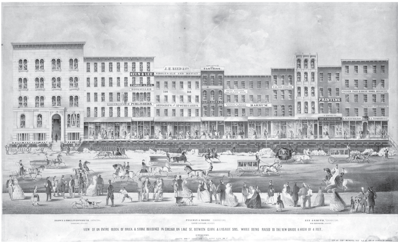
Raising a block of buildings on Lake Street, Chicago, illustration, 1857. Chicago History Museum, ICHI-059709
