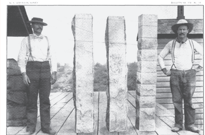
Granite survey pillars used to mark the boundary line between Idaho and Montana, 1897–98. Bulletin of the United States Geological Survey (1900)
