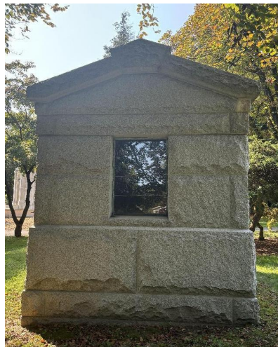
The back facade
