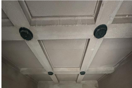
The coffered beam
