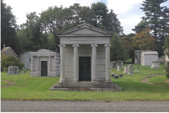
Figure 3: South East Elevation
