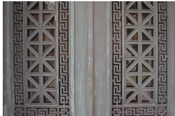
Figure 8: Bronze deterioration
