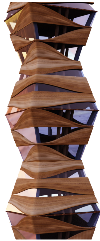
Pre-fabricated Rammed Earth Walls with Fabric formwork. Walls are formed with the combination of fabric on the front side as formwork for casting with the supports of wood formwork from remaining 3 sides. The shape after casting is bulging out, resulting in walls taking shape of fabric, which gives it an aesthetic look as well as it's properties.
