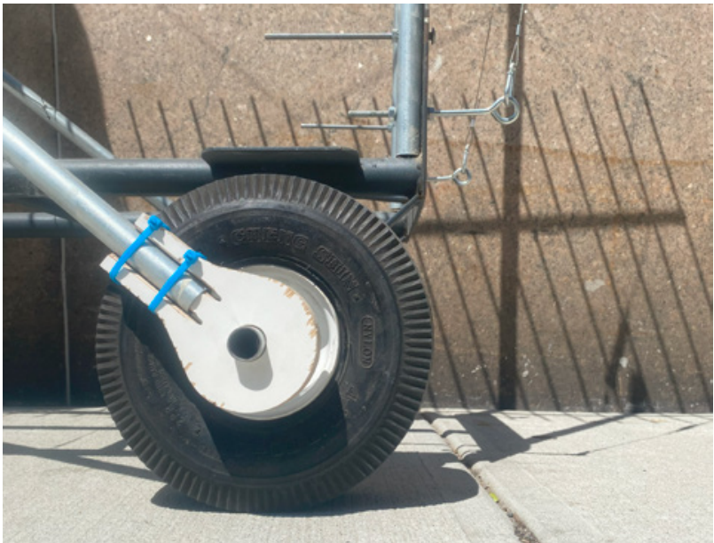
Detail showing the axle lock, column connection, and cable mounts
