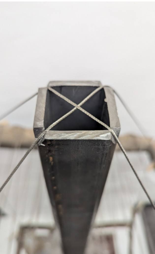
Cable grooves notched into vertical HSS
