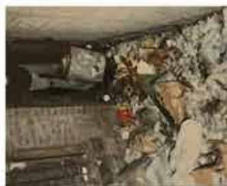
Basement and Airshaft clean-up
