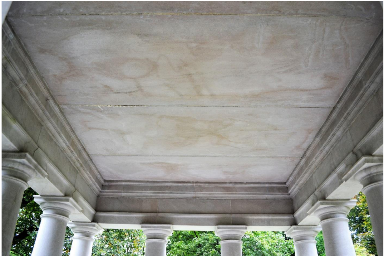
2.9 Interior view of the ceiling
