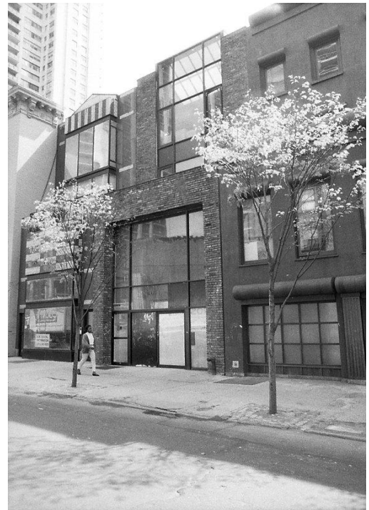
Modulightor, Inc., 246 East 58th St., New York City. Construction Photo, 1988. © The Estate of Paul Rudolph, The Paul Rudolph Institute for Modern Architecture.
