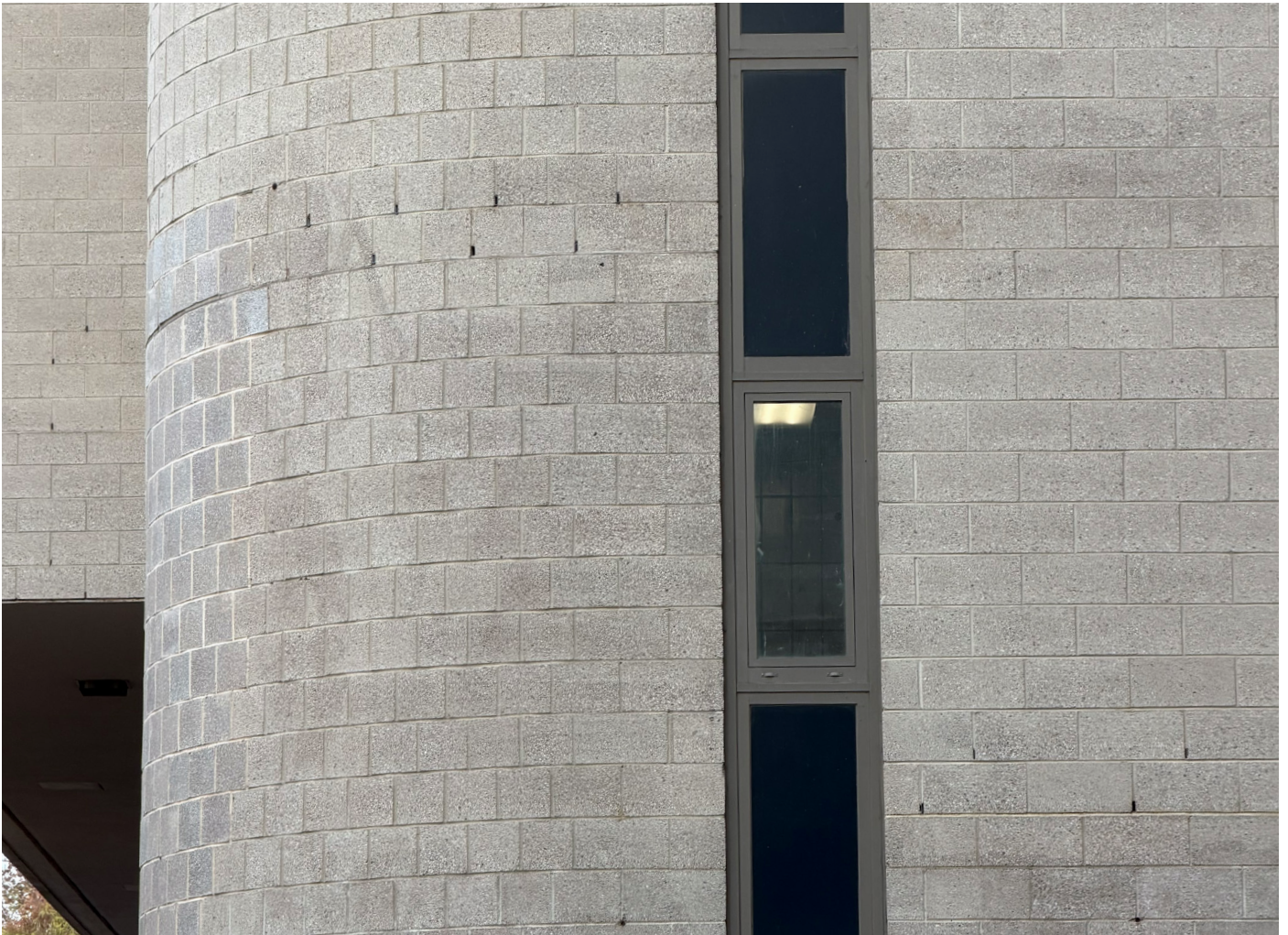
Figure 18: I.S. West facing facade, usage of CMU Brick. Source: Author
