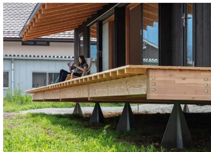
An eco-friendly house elevated on recyclable iron stilts. Akeno raised floor, Fuminori Nousaku.
