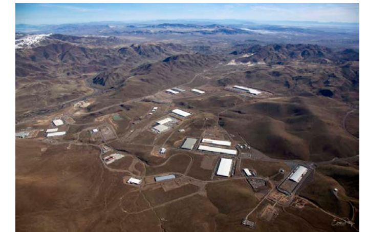
Dron over TRIC. Tahoe Reno Industrial Center
