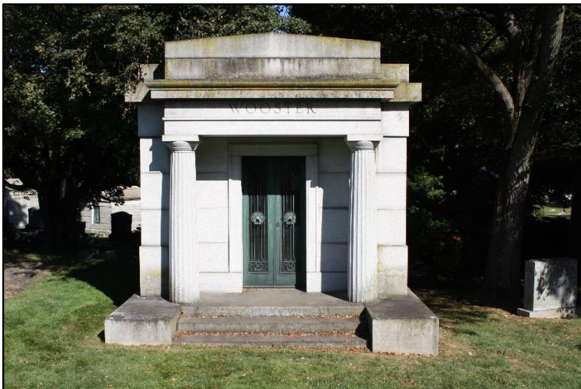
Figure 29: West elevation of the Wooster Mausoleum.
