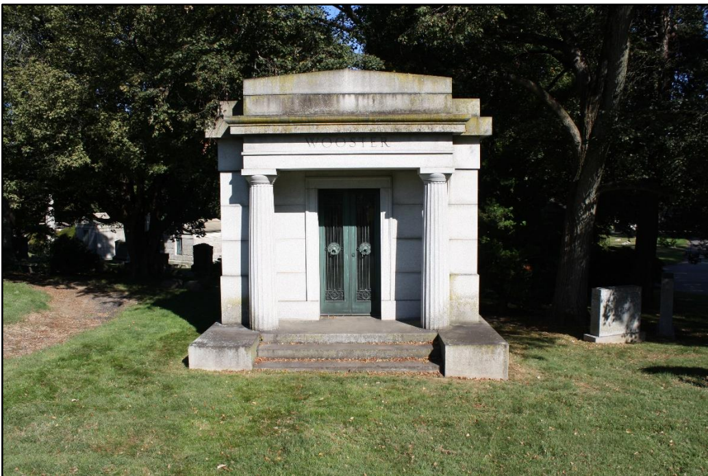
Figure 10: West elevation of the mausoleum.
