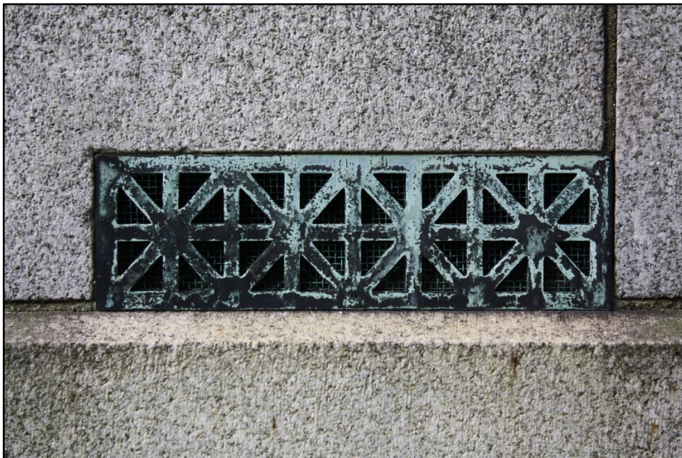
Figure 16: Close up of a copper alloy vent grille.
