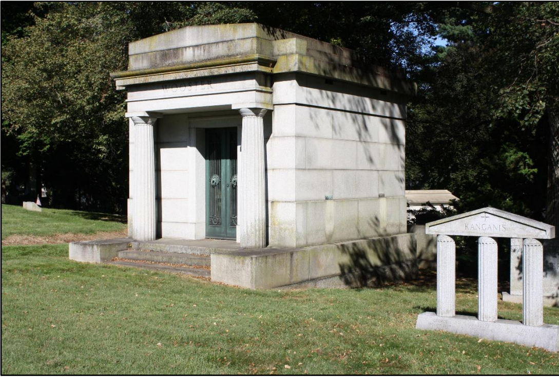
Figure 11: Skewed angle of the west and south elevations of the mausoleum.
