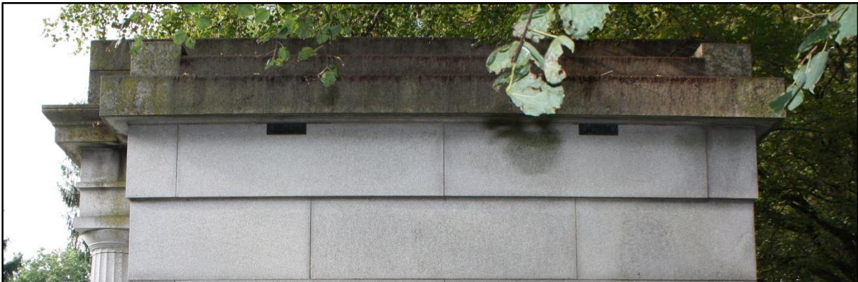
Figure 14: Granite banding as seen from the south elevation.
