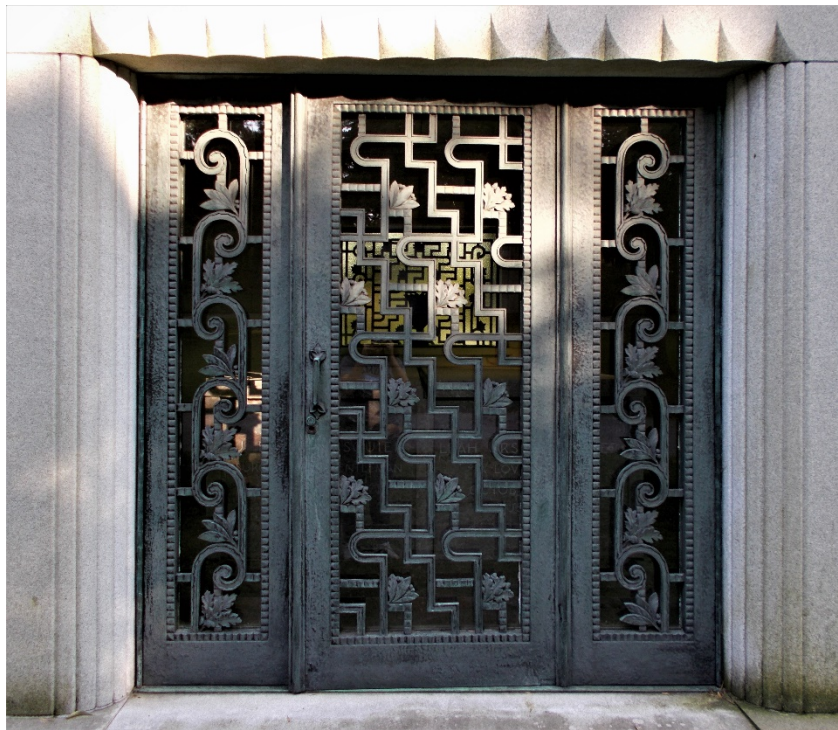
Figure 13: Reeding around front door on façade of Squier Mausoleum
