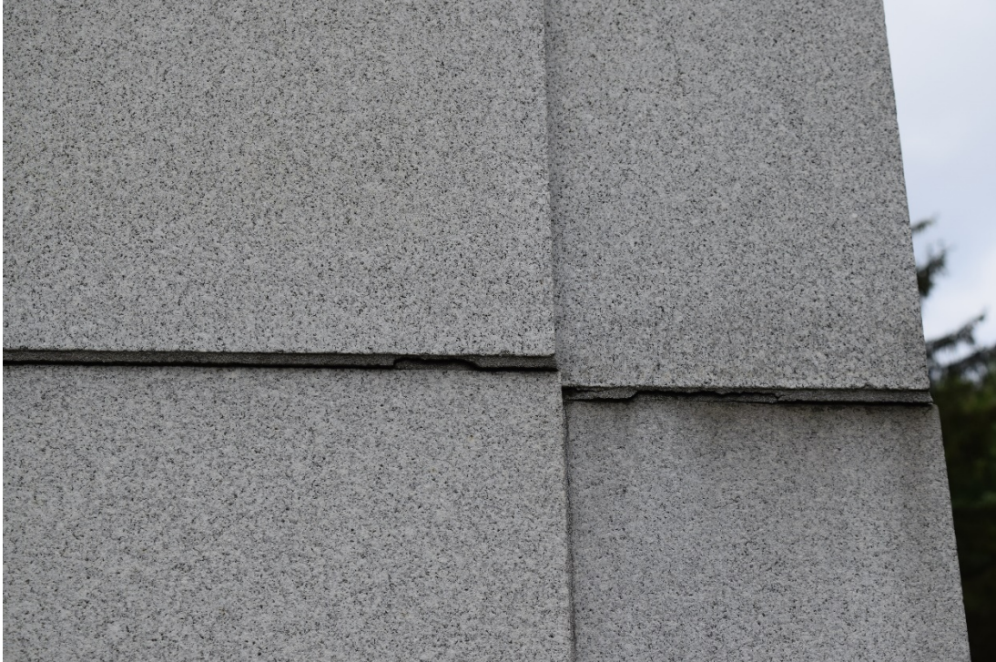
Figure 20: Repointed mortar on Southwest Elevation
