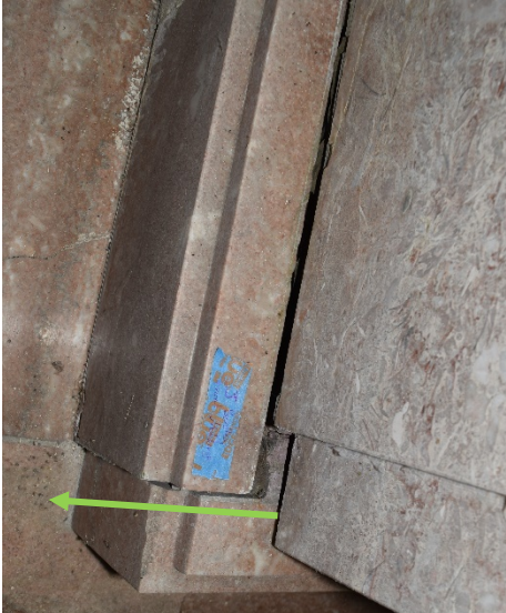
Figure 27: Displaced corner joint on J. Bentley Squier's sarcophagus
