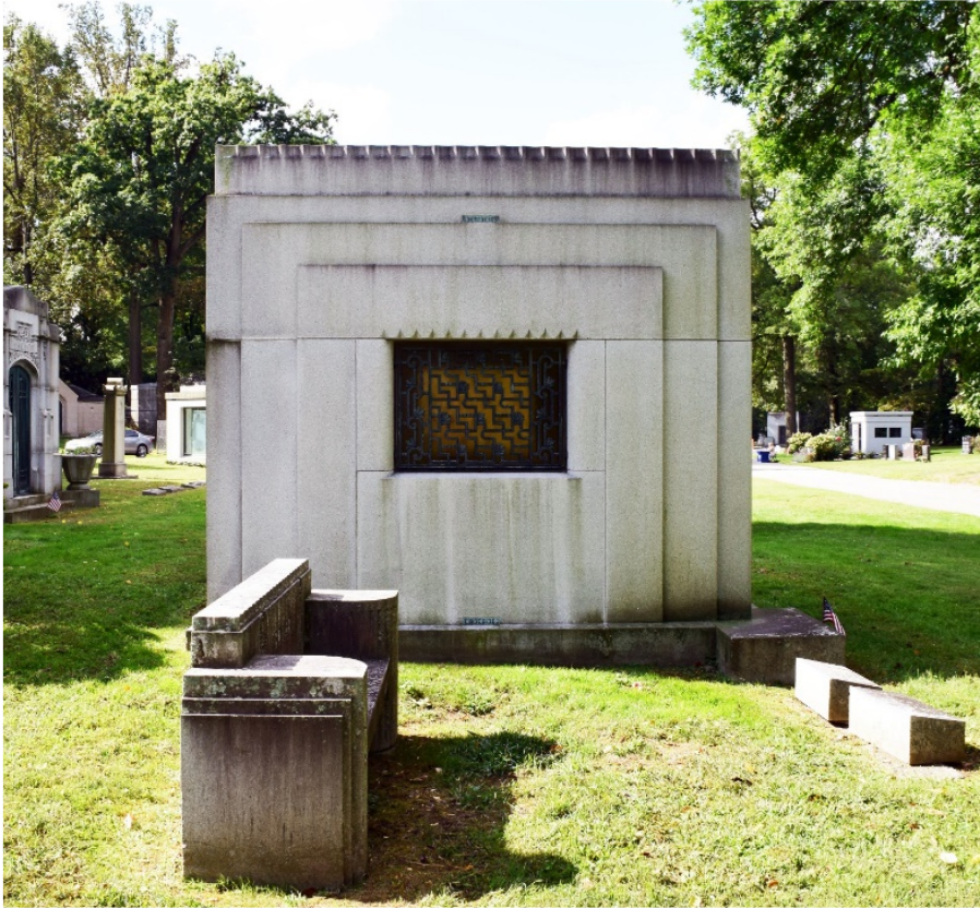
Figure 12: Side (northeast) Elevation of Squier Mausoleum with stepped protrusions
