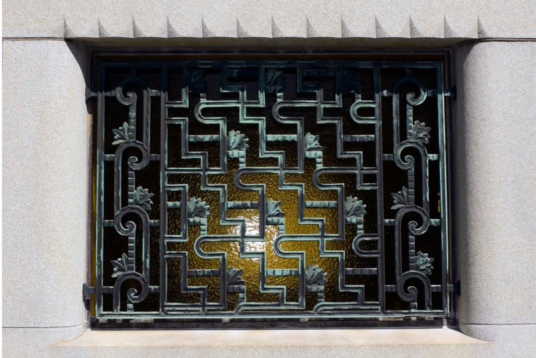
Figure 7: Close-up of J. Novelli window grille on northeast elevation
