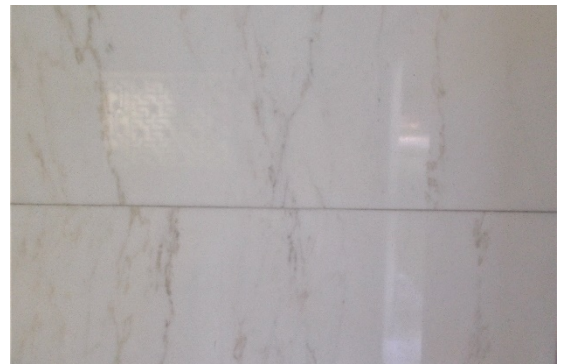
Figure 15: Sample of interior cladding on ceiling
