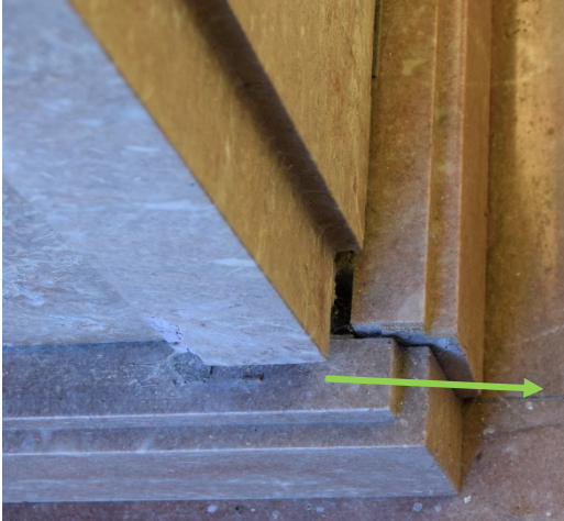
Figure 28: Displaced corner joint on Leah Ursula Squier's sarcophagus
