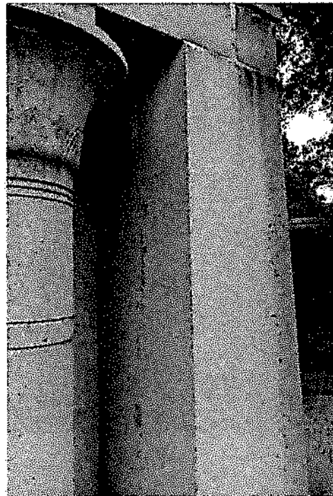
Fig. 9 Interior of front façade right pylon.
