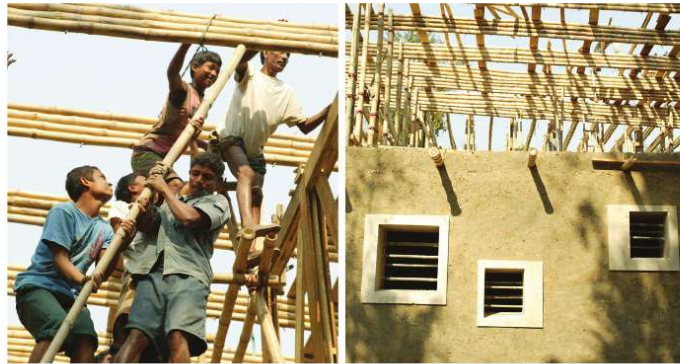
Figure 6. Construction of the METI School using community labor (no crane to lift trusses); windows are plastered with a sand-and-lime mixture. Photo by Kurt Hoerbst. ( Anna Heringer | METI School, Bangladesh (n.d.), https://www.anna-heringer.com/projects/meti-school-bangladesh/ )
