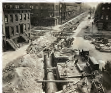
"Construction of Water Main Pipes in Manhattan," c. 1928, photograph, likely related to the New Croton Aqueduct system or city water infrastructure upgrades, New York City Municipal Archives. Accessed July 27, 2025.
