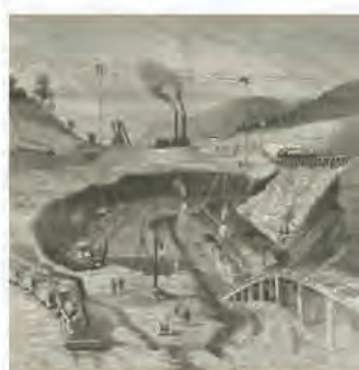
Excavation for the New Croton Aqueduct, Showing Steam Shovels and Narrow-Gauge Railway Tracks, engraving, c. 1887, Courtesy of the New York Public Library Digital Collections.
