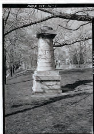
Historic American Engineering Record. Old Croton Aqueduct, Ventilator Shaft No. 9, Van Cortlandt Park, Bronx, New York, HAER No. NY-111-1. Photograph by Jack Boucher, 1978. Library of Congress Prints and Photographs Division. Accessed July 27, 2025.
