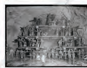
"Drill Gang at Work in Tunnel," The Myrian and Ira D. Wallach Division of Art, Prints and Photographs: Photography Collection, The New York Public Library Digital Collections, accessed July 27, 2025.
