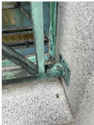
Image 12: Blue Rust on the Window
