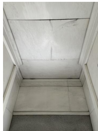
Image 10: Water stain on the Roof
