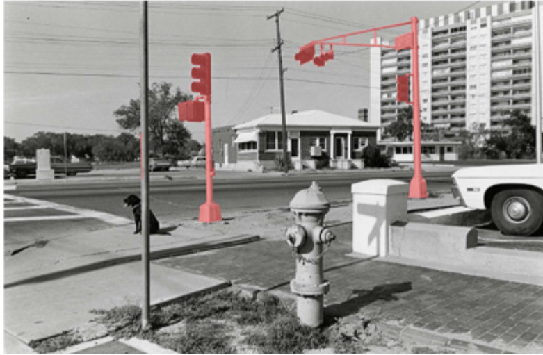
Optic Signals, Galvanized, Steel. Cantilever
