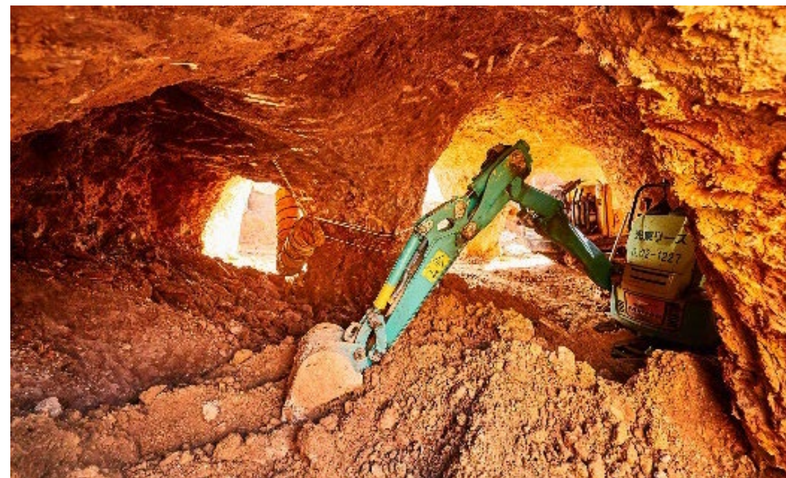
Underground restaurant under construction.
