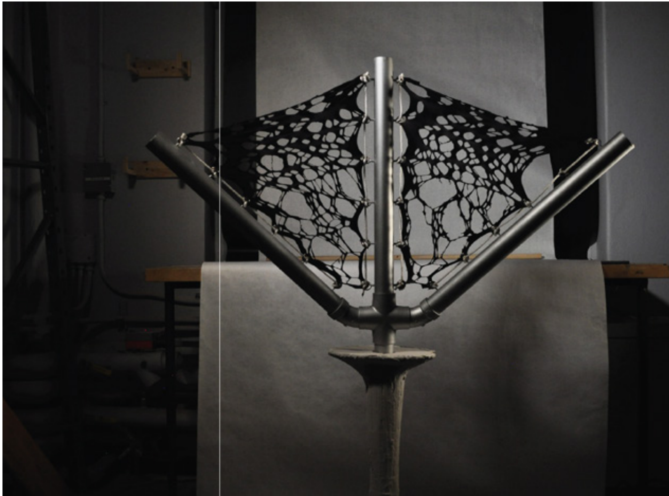
Simple assemblies with grommets fabric and cables permit the maintenance and repair of the memorial's skin.
