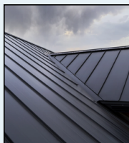
Standing Seam Metal Roofs
