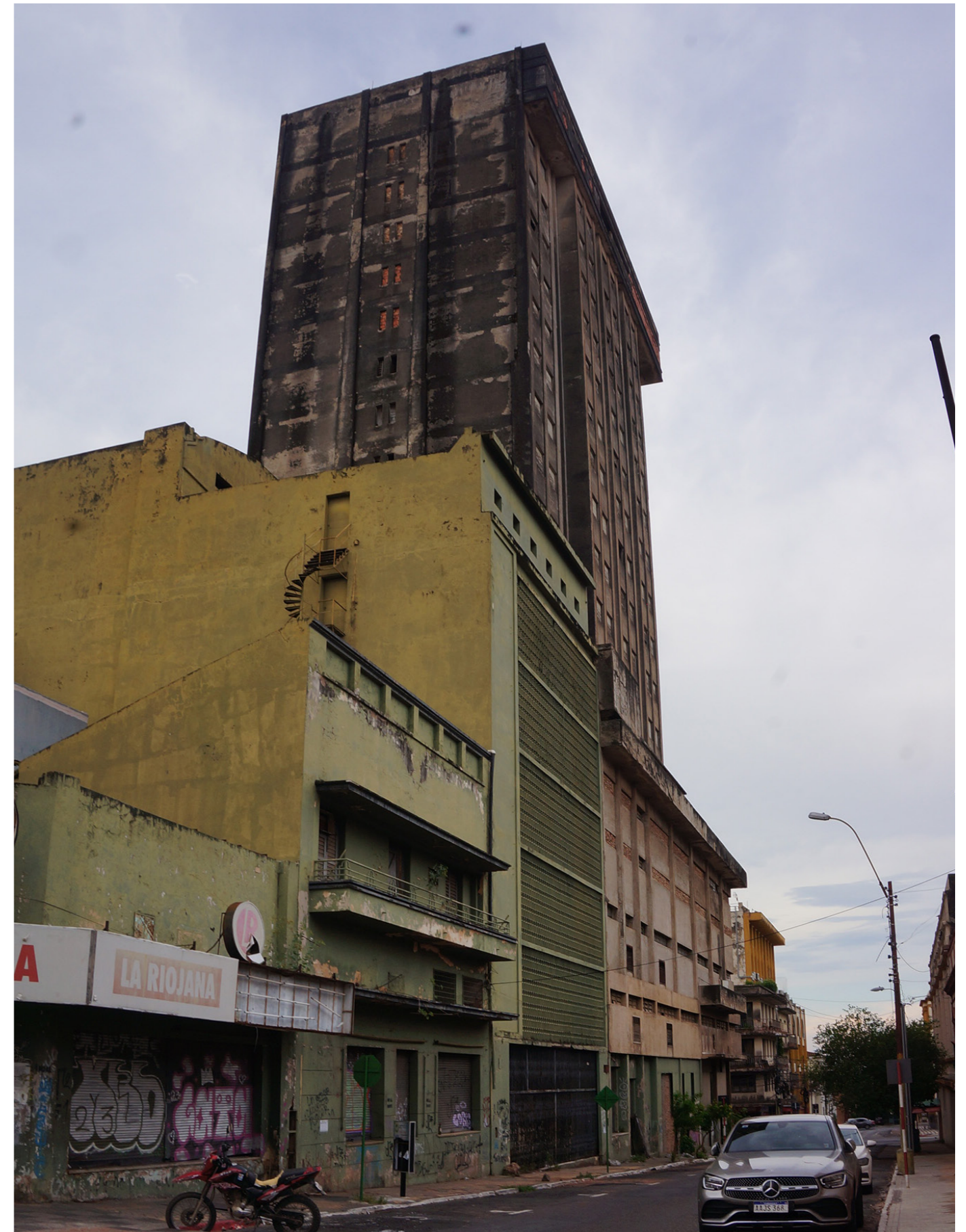
Fig.27. Vacant building in the Historic Center of Asunción
