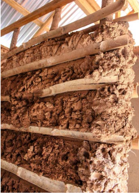
Exposed Wall at Adako-Jachie
