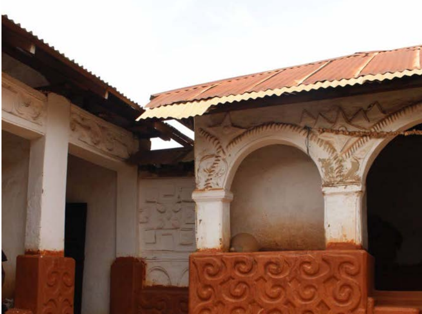
Replacement Metal Roofing at Asawase
