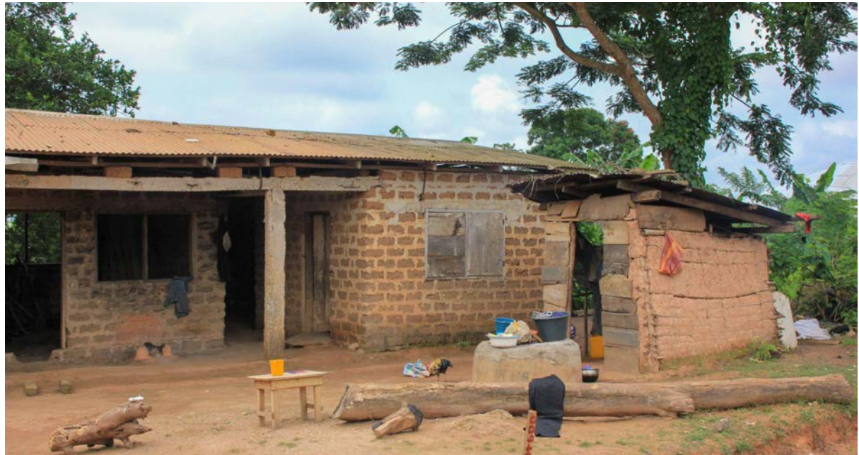
Earth block house and tadan building on the road to Patakro Image by Daniela Martínez
