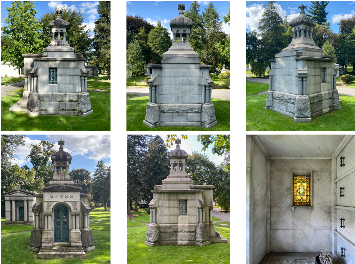
Figure 6. Photographic elevations of the Gross-Noll mausoleum, and an interior view showing the stained glass window and marble finishings.
