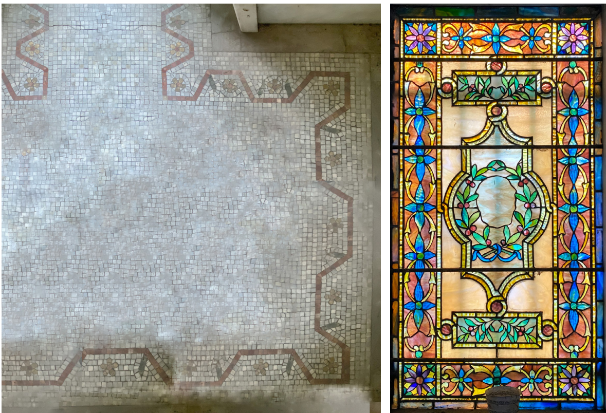
Figure 9. Left: Mosaic floor is made of Marble and Terracotta tiles following geometrical and flourish motifs. Right: East facade Stained glass window. East facade and West facade windows share the same pattern design.
