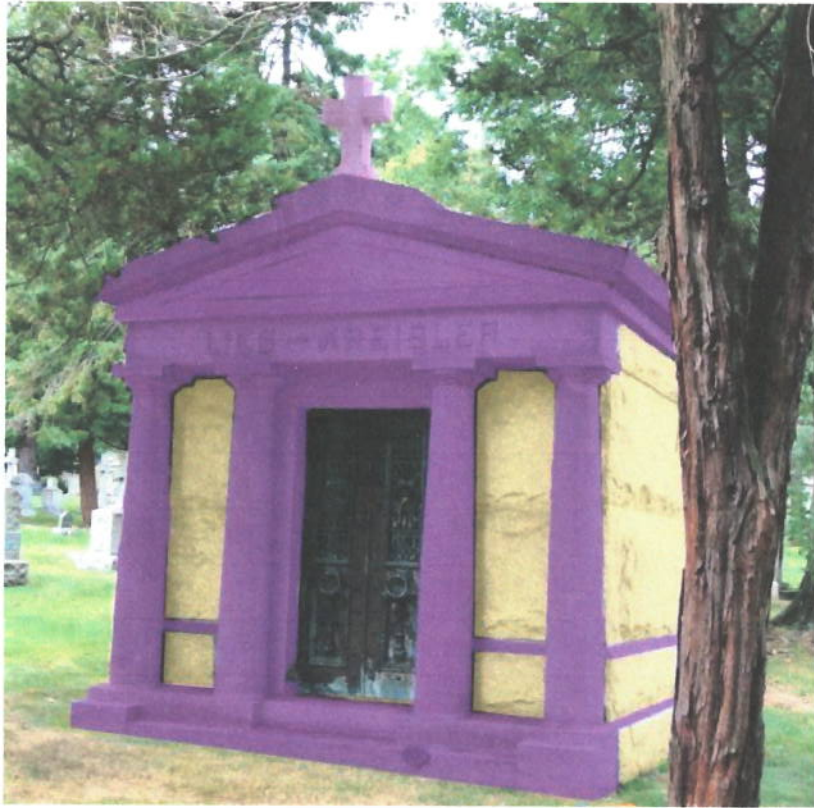
Figure 3: "rock-face" finish of granite body and smooth finish of granite entrance, portico, and pediment
