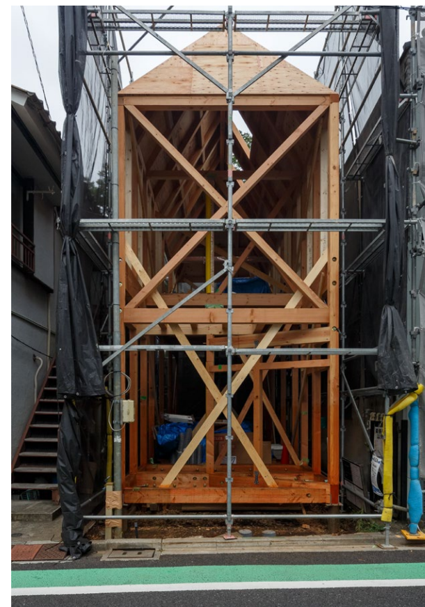
Piles and Pointed Roof: The Wooden Structure,
